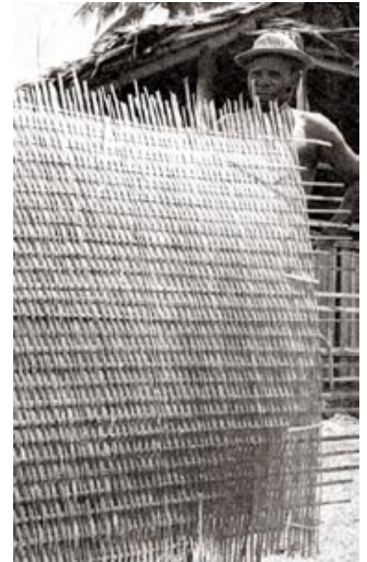
Left: The walls of this timber framed experimental structure are lined with Sago woven mats manufactured by a locally developed handloom.
