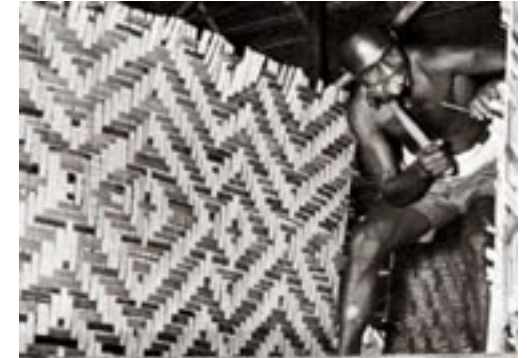
Building components in traditional construction were generally put together by tying sennit. This is now being replaced by nails which are manufactured locally in Papua New Guinea.
