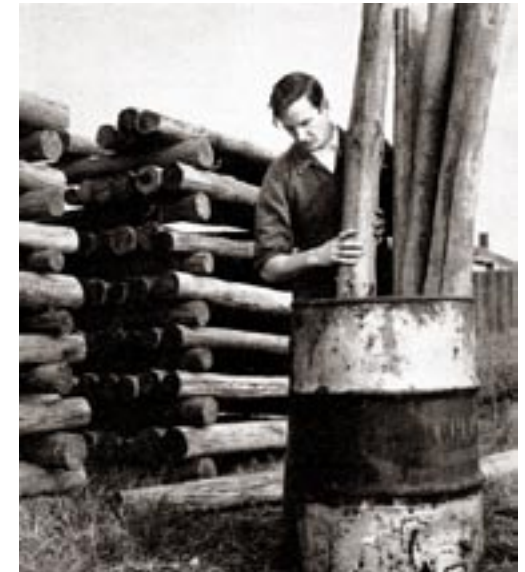
Dip diffusion is a suitable method of treatment for small amounts of timber.
